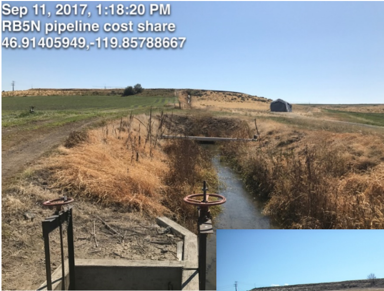
Jan 5, 2018 at 12:41:01 PM RB5N pipeline
